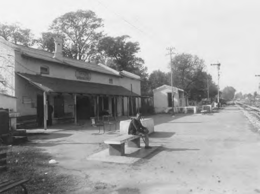
The Harawala railway platform near Manjri Mafi
