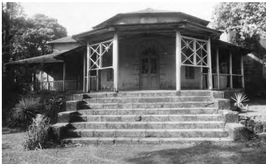
The stairs to the drawing room of Florence Hall
