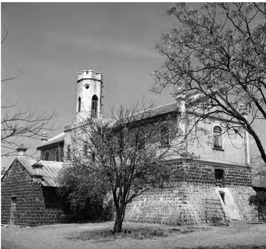
The entrance to the East Room of the converted water tank
